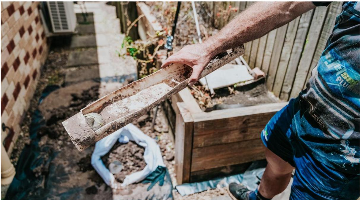
Over 90% of homes we inspect have either cracked, broken, collapsed or tree root infiltrated pipes and drains. This issue can cause “undermining” (if you’ve ever seen a
